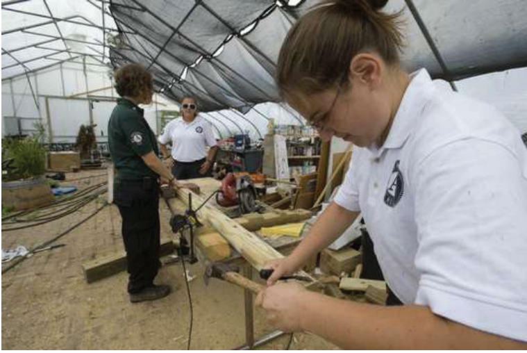
Avi Steinhardt/Courier-Post 6/10/09 -- Americorps volunteer Noel DiDomenico (right, front) chisels out a notch in a fence railing with the help of fellow volunteers team leader Joareyn Hill, (left, back) and Sadie Stone at the Camden Children's Garden.
